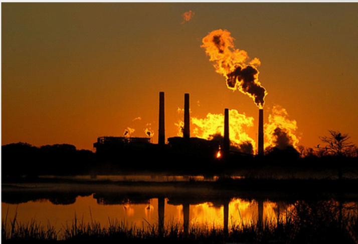
The W. A. Parish Plant, pictured above, is the largest coal plant in Texas. Texas has more coal-powered plants than any other state.
